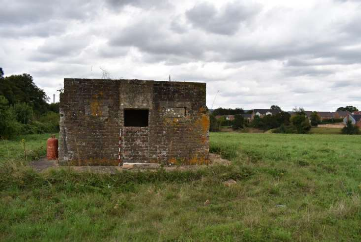
Plate 11: View of the entrance to the Pillbox (facing NE). Scale 1m
