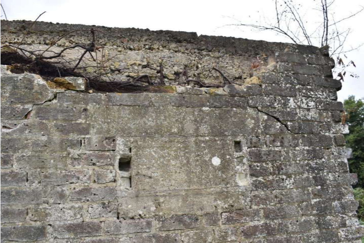
Plate 17: Close up of the shuttering and concrete on north eastern side (Facing W).
